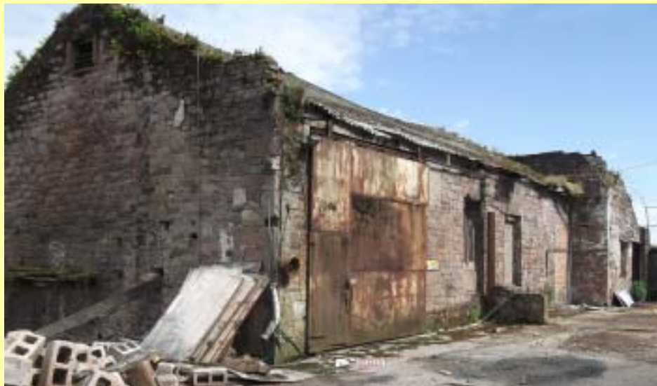
2012 saw the demolition of a sizeable collection of vernacular buildings off Albion Street in Whitehaven, which will be replaced by an office development
