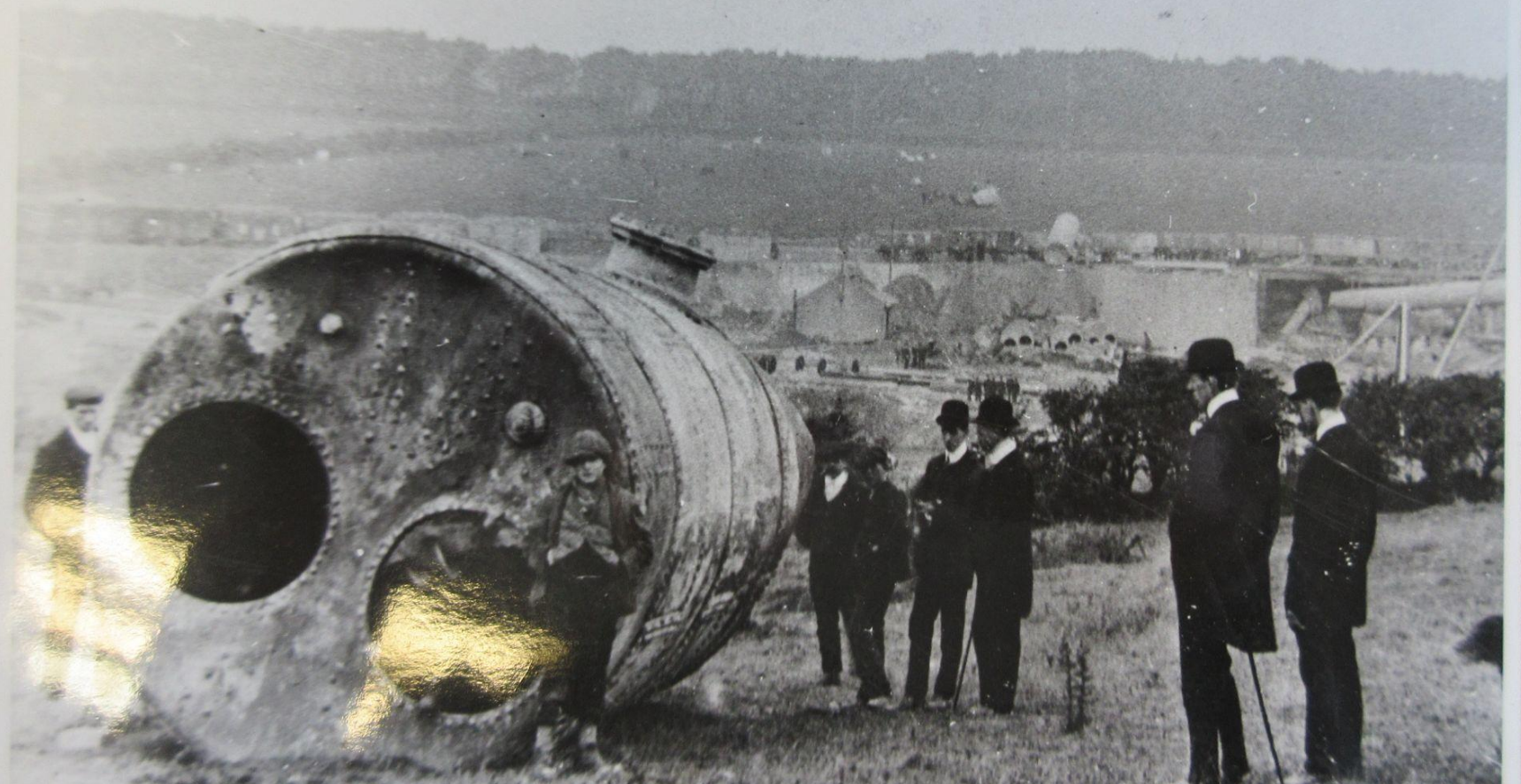
Roller down 500 yards at Distington Iron Works Sept 18 - 09.
