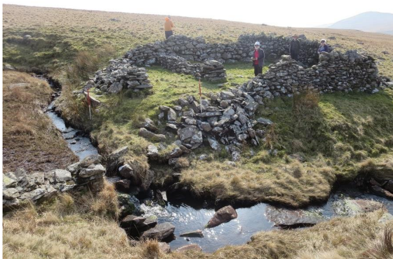
WF21-05 Dam and original pool size; Freeze Beck – SD 18963 96307
